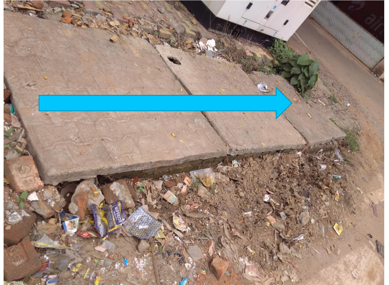
Pre-existing drainage line to connect the proposed drainage
