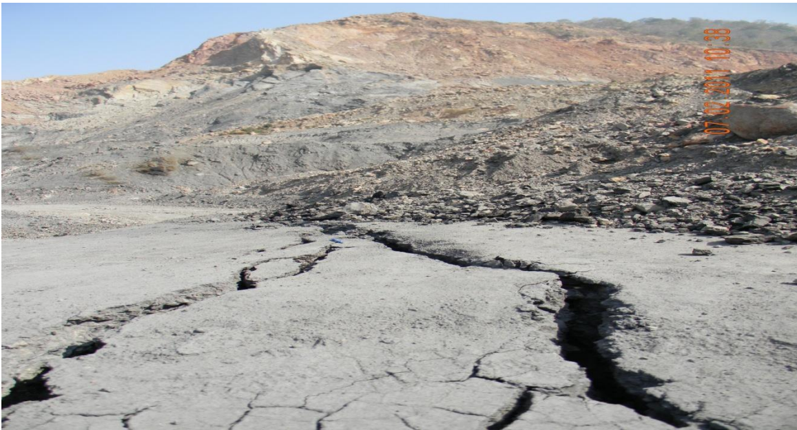
Exposed fault plane in Failure of Jhingurdah ocp (Singrauli coalfield)
