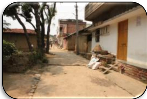
Fig. 7.16: Internal roads (PCC roads)
