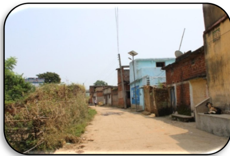
Fig. 7.32: The solar street lights
