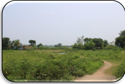
Fig. 7.49: Partially paved road from Kandra to Labudih
