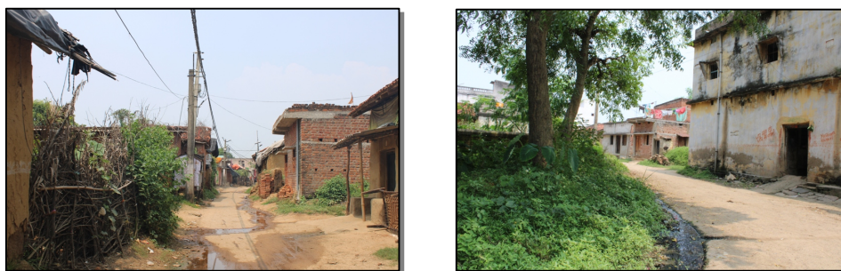
Fig. 6.10: Existing condition of drainage in Kandra GP
