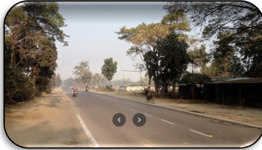
Fig. 7.45: Raghunathpur - Chas Main Road
