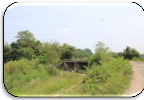
Fig. 7.17: Road (bituminous) which
