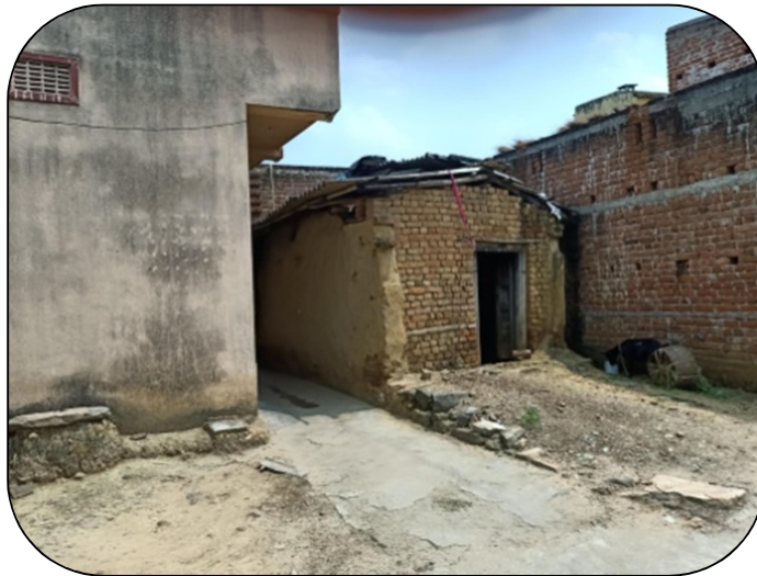
Fig. 5.13: Houses in Kandra GP with temporary roof material
