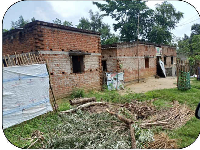
Fig. 5.12: Houses in Kandra GP
