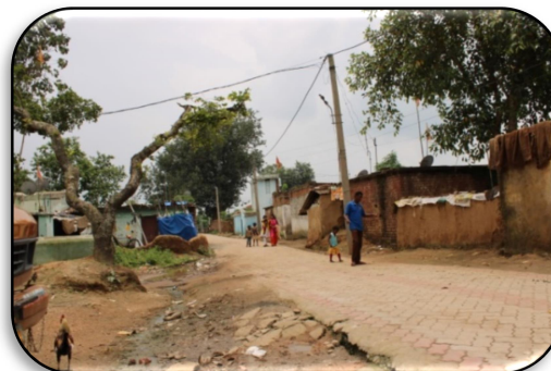
Fig. 7.13: Paved road in the GP
