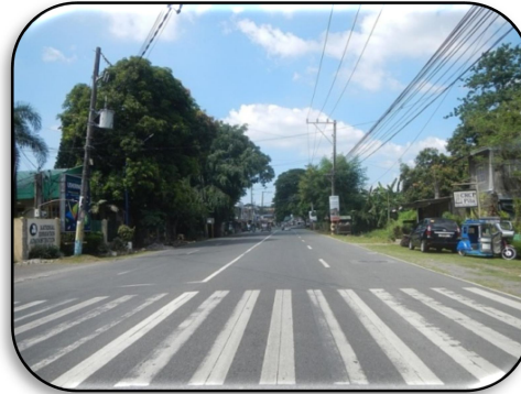
Fig. 7.47: Zebra crossing at NH
