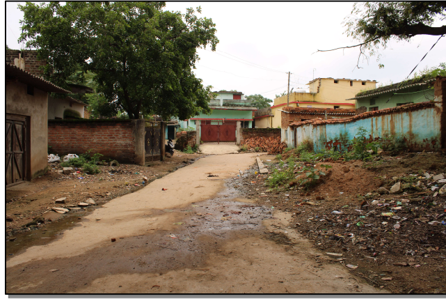
No drainage along the PCC Roads the southern and western boundary
