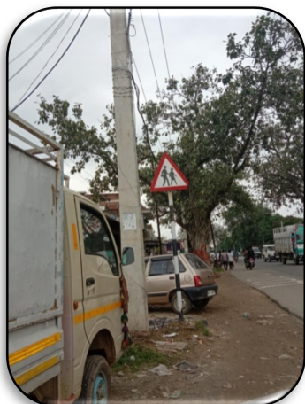
Fig. 7.20: The signage is inappropriately placed
