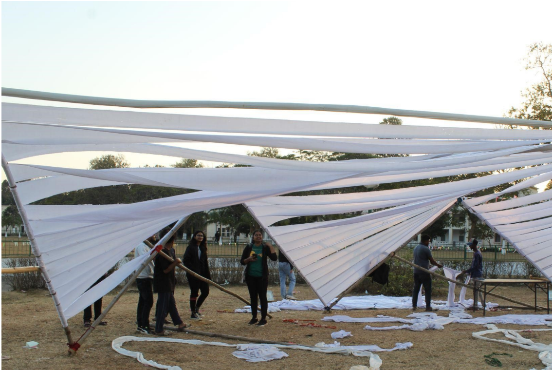
Pavilion construction in process.
